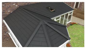
Chosen tile is added ensuring weathertightness and the gutter and external trim are secured in place.
