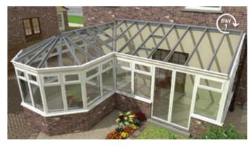
The aluminium rafters, ridges and wall plates are fitted and the spider arms are secured to the spider bracket.
